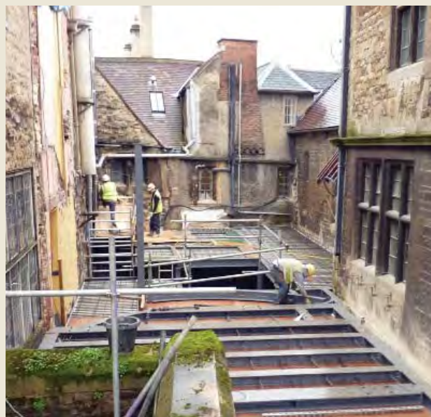
▽ The Project Q construction yard in New Quad
