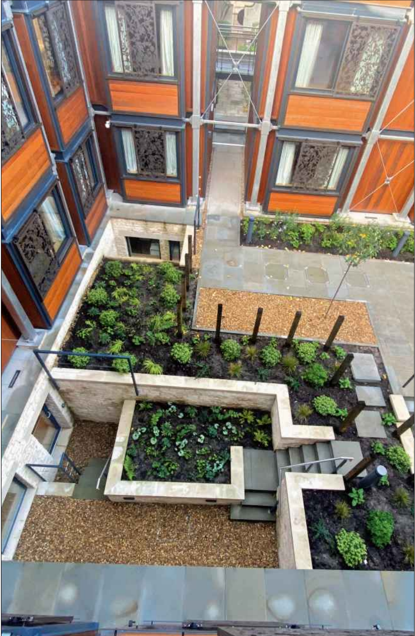
A view of the courtyard from the room.
