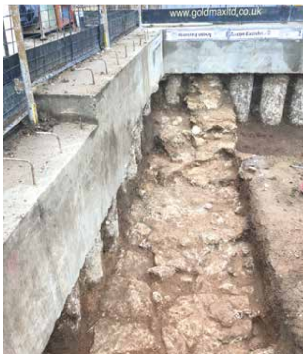
The limestone wall foundation unearthed at the site
